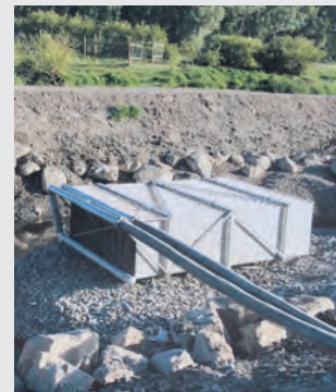
The energy savings from this heat exchange unit could be nearly 100,000kWh annually making the total carbon reduction of 74.4 metric tons. That is the equivalent of taking 15 passenger vehicles off the road each year.
