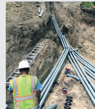
Because the high-capacity power cables and fiber optic lines were buried, they will not block views of the mountain landscape.
